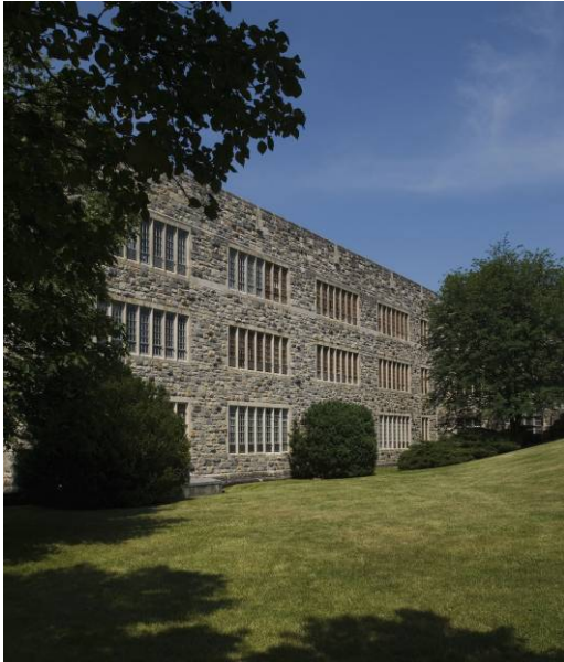
Figure 10. Norris Hall Classroom Windows, Grassy Side
