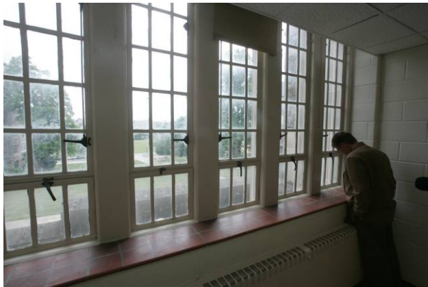
Figure 11. Typical Set of Windows in Norris Hall
